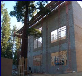
ORG-Exterior Masonry Walls-South West
