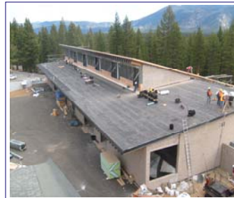
CTE Roof and South Wall
