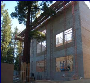
ORG-Exterior Masonry Walls-South West
