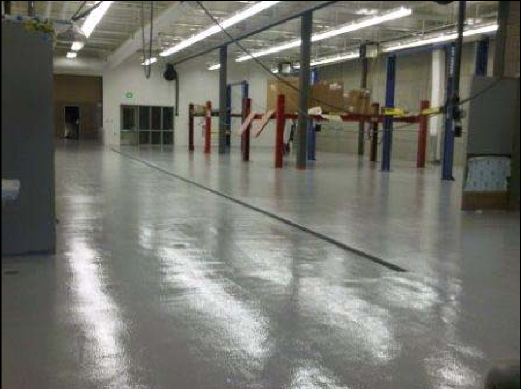
3/15/10 – CTE Lift and Alignment Bays
