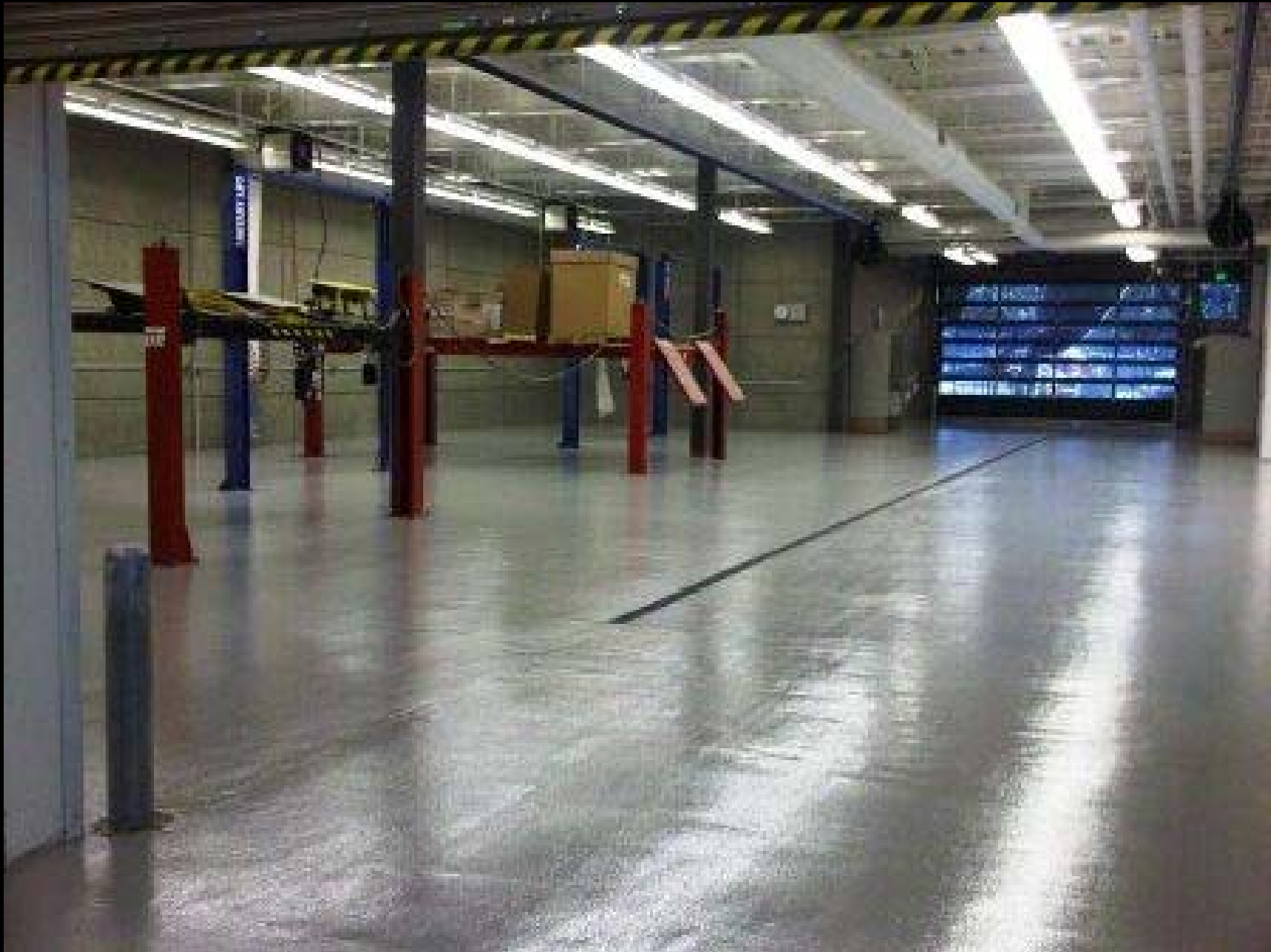
3/15/10 – CTE Auto Shop and Entry Door
