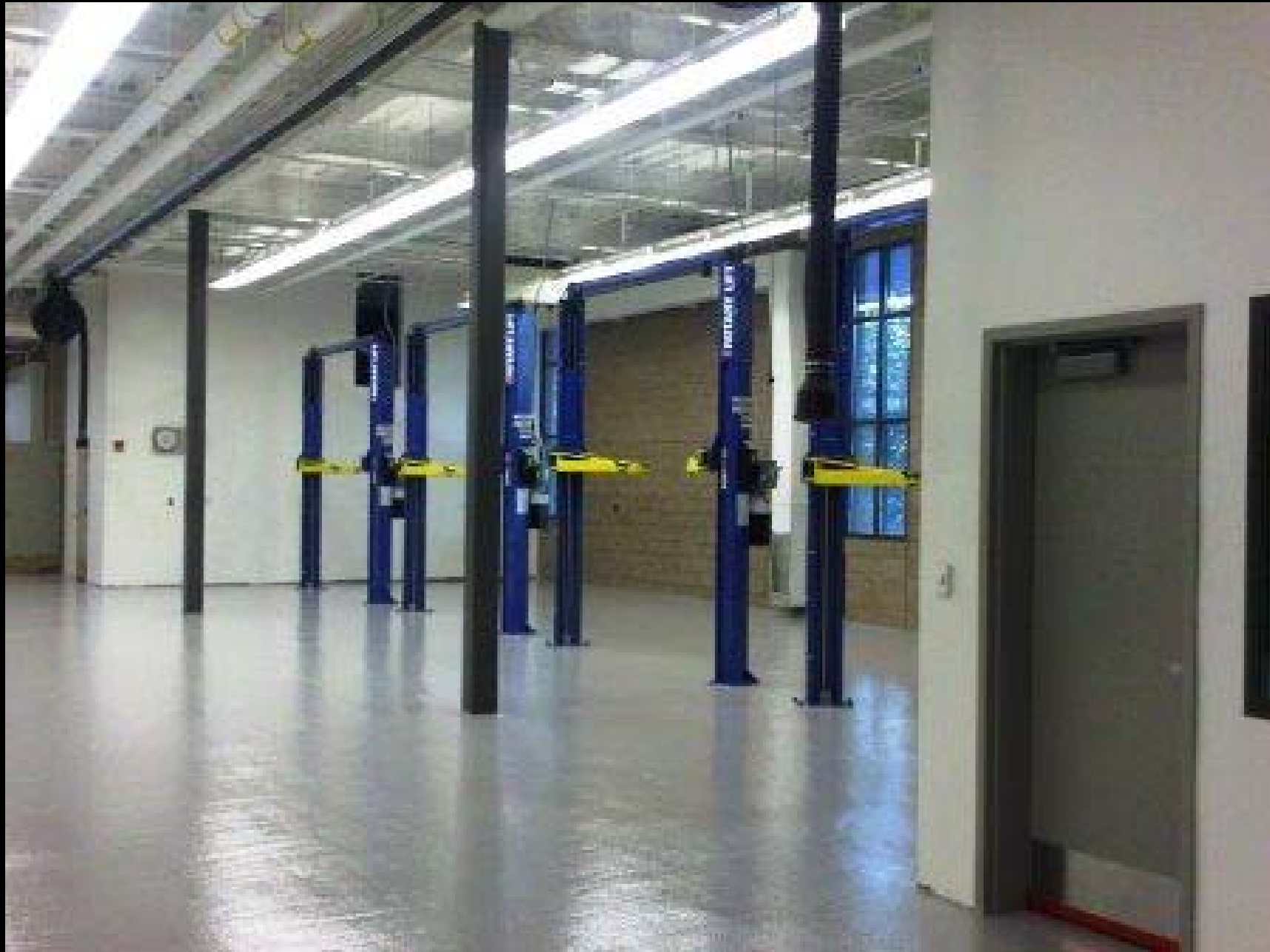
3/15/10 – CTE Auto Maintenance Bays
